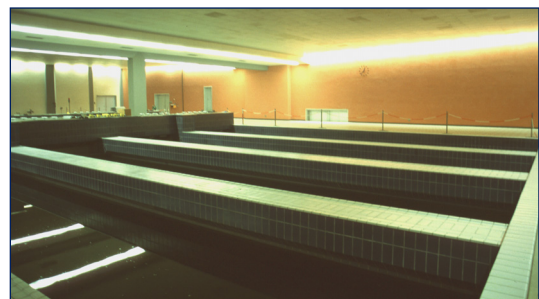
Rapid Sand Filtration – The first purification step in the groundwater recharge plant "Langen Erlen".
